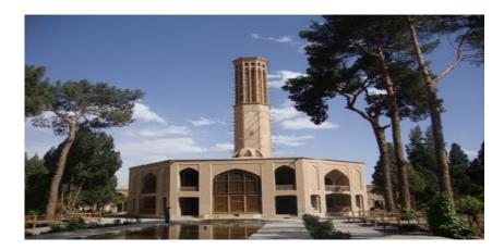
Wind towers which are used for ventilation on the roof of the house is built. Deflector as well as water reservoirs and opening mines make for ventilation. In homes cool air from the windward, the primary type of air conditioners is the ground floor rooms or basements will be sent. Deflector elements and symbols of Iranian architecture, but today are used in many Middle Eastern countries.
